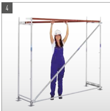
Mount decks, align scaffold bay perpendicularly to guard rail and frame using spirit level.
