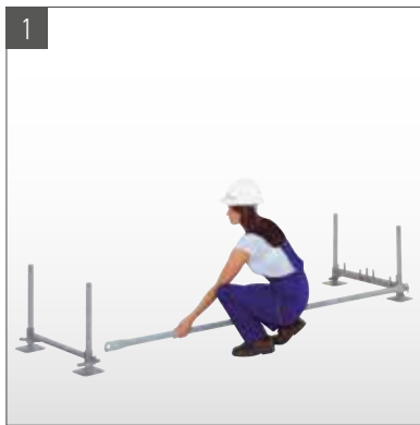
Set up the base jacks, attach base transom, mount guard rails (only in the diagonal bay).
