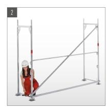
Mount vertical diagonal brace, install horizontal brace (only in the diagonal bay).
