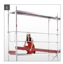
Mount assembly frame and decks of the next layer and hang diagonal, guard rail and toe boards.
