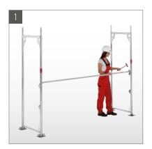
Set up the base jacks, attach assembly frame and connect the guard rails.
